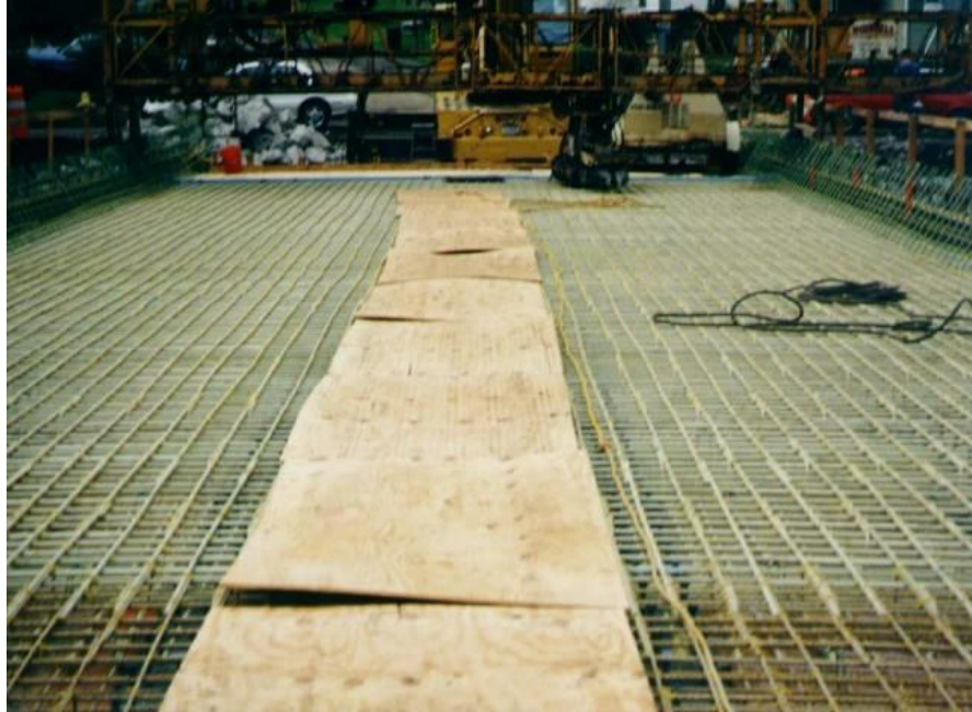
1996 – Buffalo Creek Bridge – 54 m (West Virginia, SUA)
