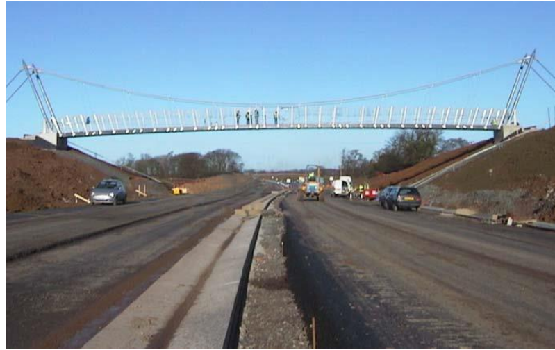
Pedestrian Bridge from COMPOSOLITE panels (Shropshire, Scotland)
