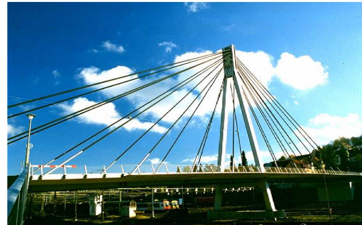
Storchenbrücke, 1996 Switzerland (124 m deschiere)
