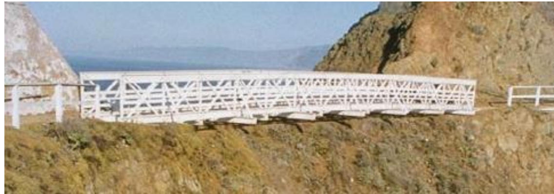
Historic Trail Bridge with 21m opening
