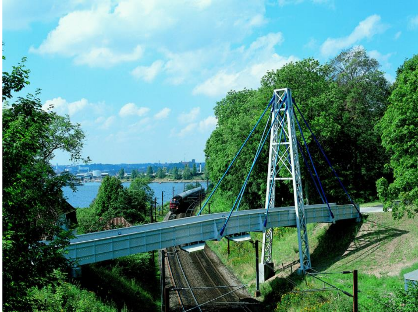
The Fiberline bridge in Denmark
